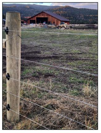
This electric fence built in 2023 was designed to keep bears away from attractants like livestock feed that are typically stored in sheds and barns.
