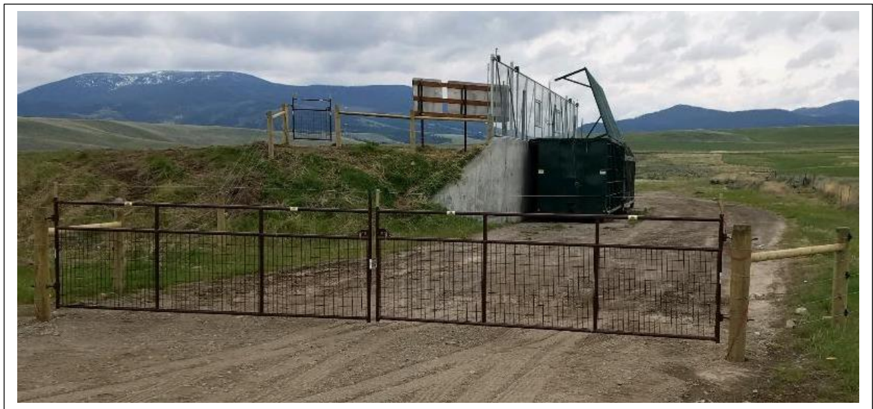
The new Helmville Transfer Site electric fence. Photo by Eric Graham.
