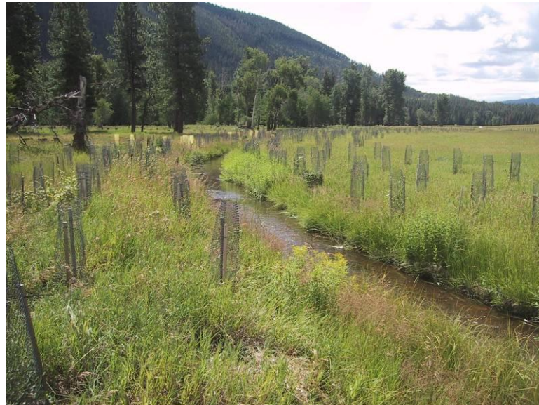
Photo 41: Upper Rock Creek Photopoint 5: upstream end of Reach 3 (Salmon Creek from below the county road to the confluence) looking downstream. During channel reconstruction in 1998, this channelized reach was left largely untouched, and therefore is somewhat incised. The remains of the old dike are visible on the left bank; this posed problems for planting close to the stream.
