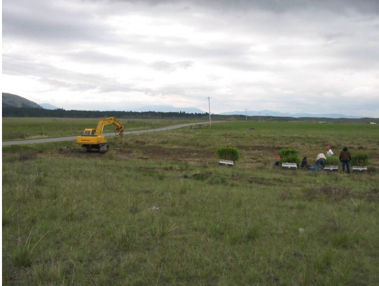
Photo 22: Planting the Lower Rock Creek site in May 2005 using PVC-containerized plants and the excavator-mounted expandable stinger.
