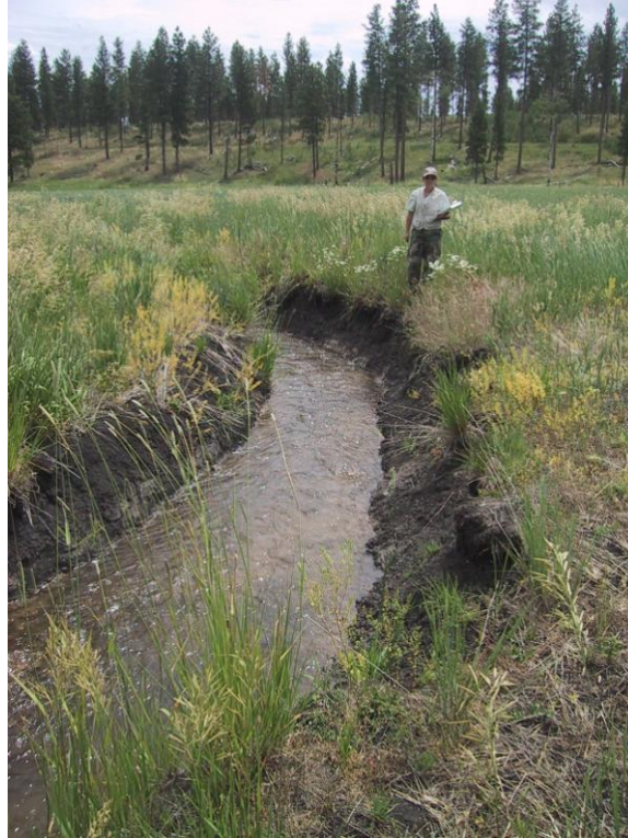
Photo 5: Incised section on newly-constructed channel. The planting group at this location has all died, and the protectors and mulch mats were removed by maintenance crews. Note vegetation community dominated by upland pasture grasses and annual weeds.
