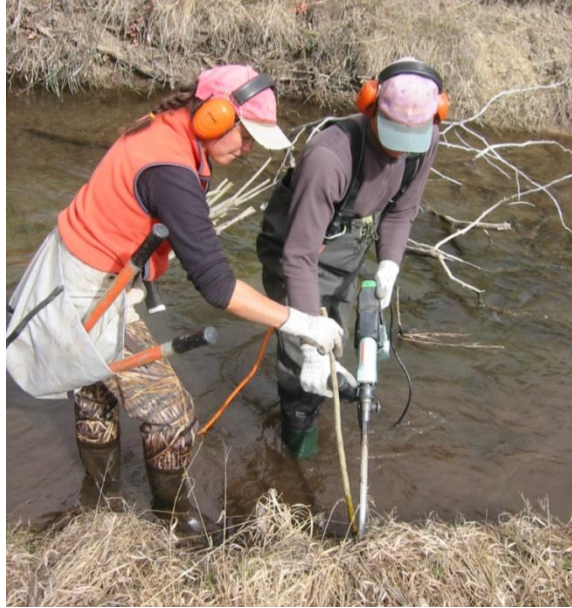
Photo 31: Installation of 30” willow cuttings using an electric hammer.
